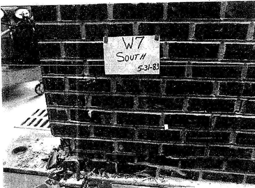
b) Bearing failure in wall W7 (brick side)
