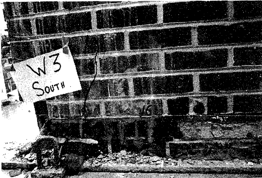
a) Bearing failure in wall W3 (brick side)
