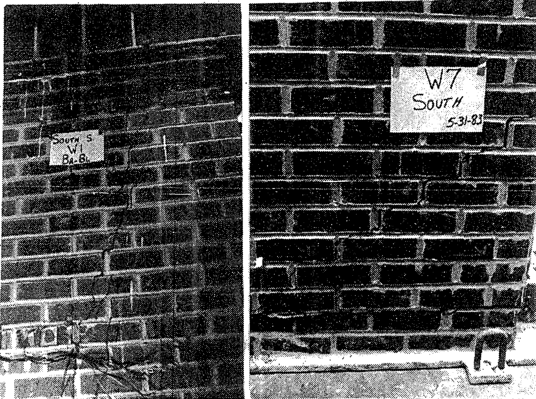
a) Diagonal crack in the brick b) Stair-step crack
